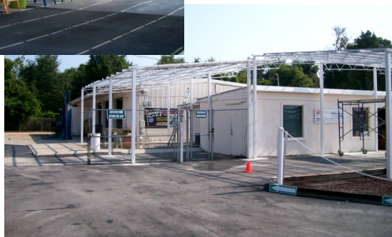
Construction Phase August 2011
