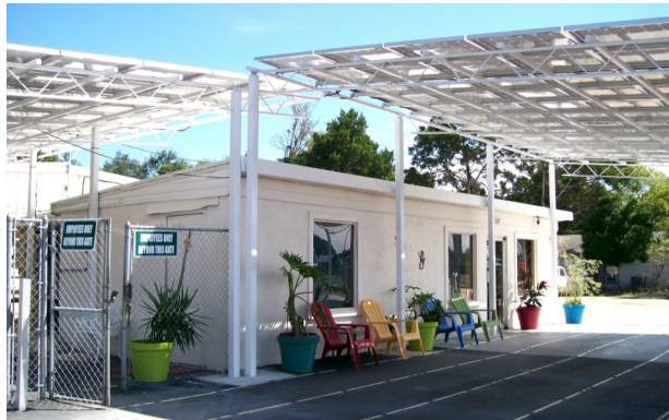
The Final Product 17 kW Grid Tied Photovoltaic System September 2011
